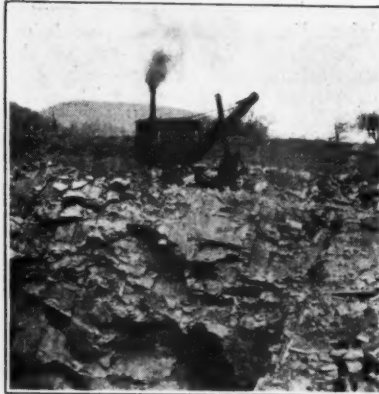
Steam Shovel Stripping 90 Feet Above Working Level.
